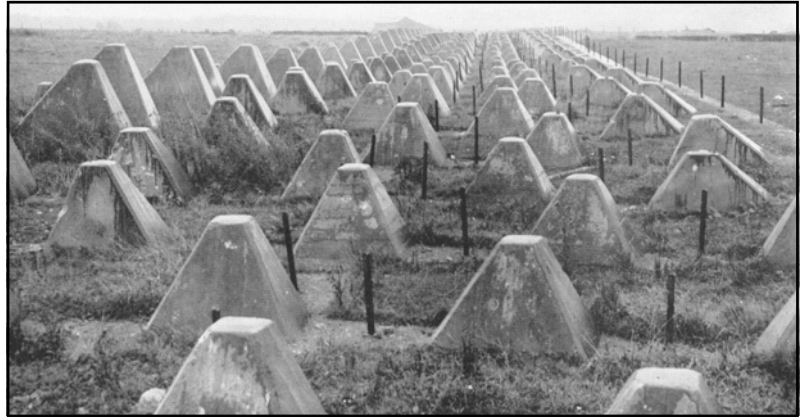
The Germans set up "Dragon's Teeth" in an effort to slow the Allied pursuit. These concrete obstacles were easily eliminated by direct fire from the tanks.
